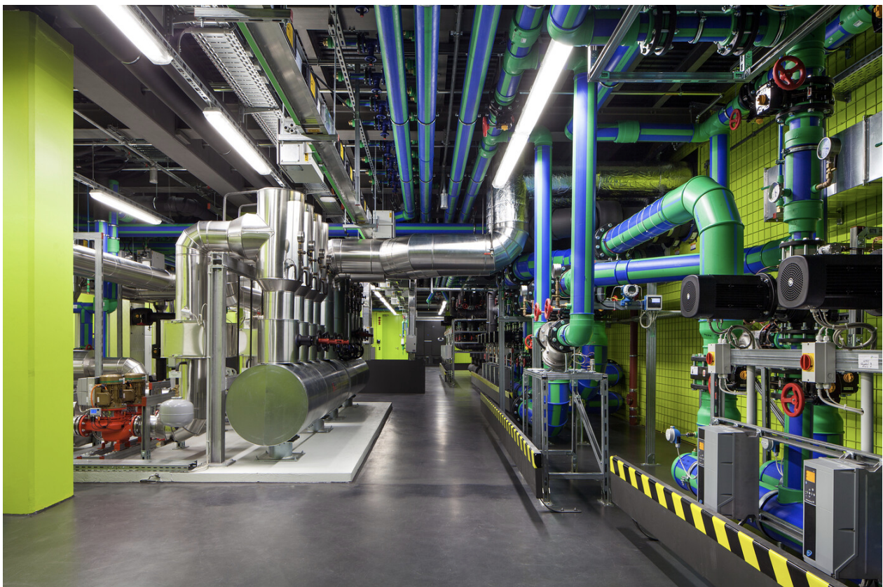
Cooling infrastructure of the server rooms of ZIH, TUD (2022). Photo: Robert Gommlich/© Courtesy of TUD's Center for Information Services and High Performance Computing (ZIH).
